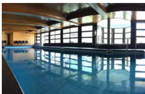
Beheiztes Hallenbad, 29°, 6,5m x 12,5m Heated indoor pool, 29°, 6,5m x 12,5m
